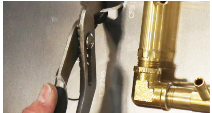
Photo 2: Breaking the Knockouts
